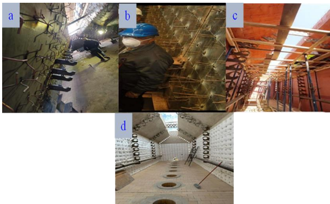
Fig. (4): Refractory lining installation sequence for furnace sections: (a) Section C wall with completed metal anchor reinforcement grid: (b) Close-up of the welded anchor pattern on the Section C wall: (c) Installation of wooden formwork inside Section B prior to casting: (d) Section B after formwork removal, showing the finished refractory lining.[1]
