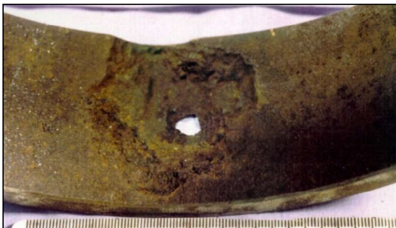
Fig.(7) Corrosion pit in a sour regime
