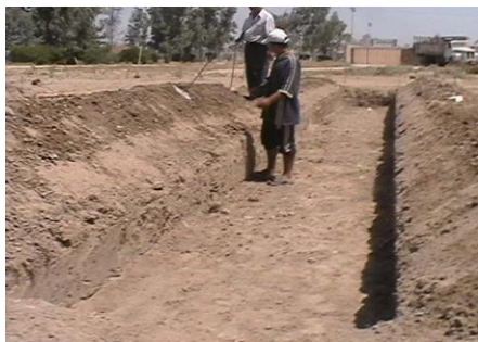
1 st . Cell during construction 1 PPP06/2007 Photo ( 1)
