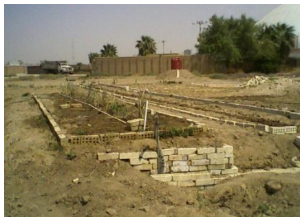
1 st & 2 nd .Cells after construction and reed plantation 08/2007 Photo (2)
